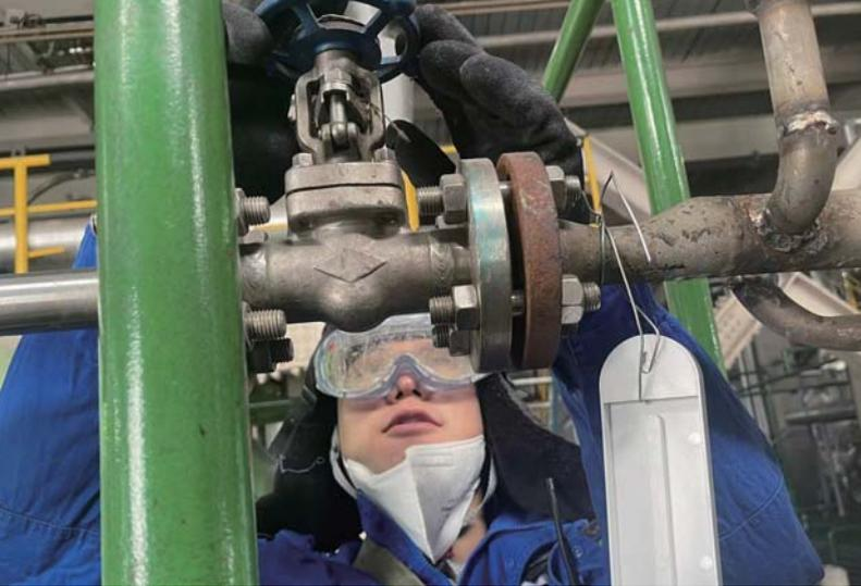
Adjusting refill valve of ammonia pump tank
