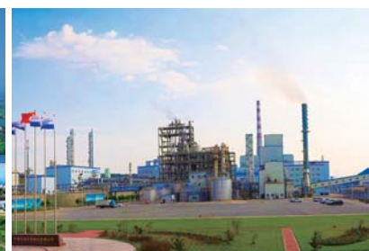
The production facilities in Heilongjiang
