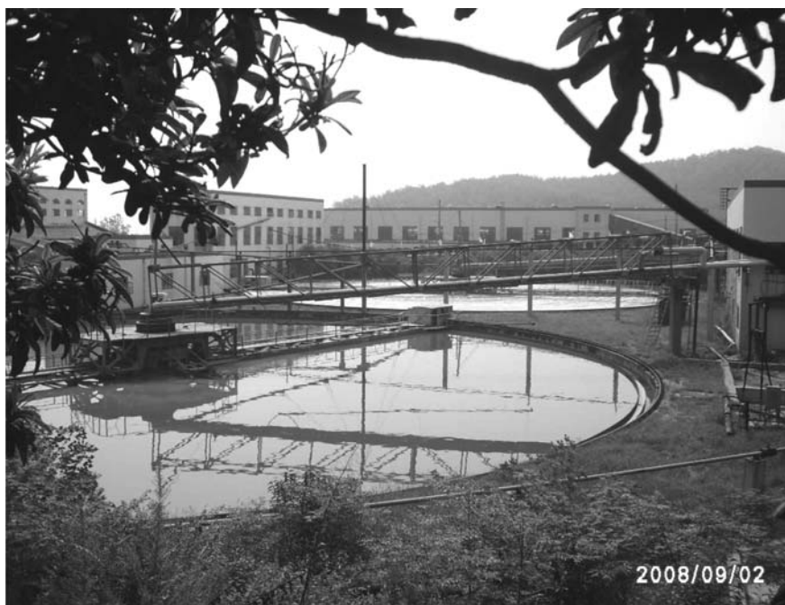
Figure 3.21: Dayukou — Phosphate 50m Diameter Thickeners
