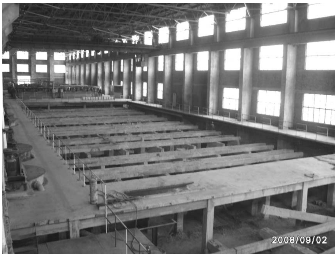
Figure 2.11: Wangji — Phosphate Plant Floatation House with Obsolete Cells Removed
