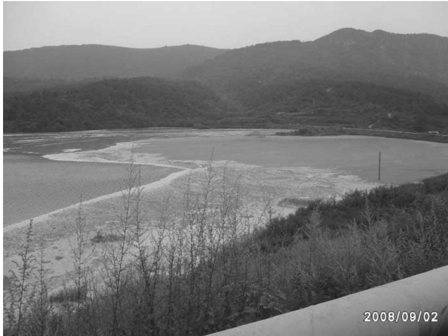
Figure 3.22: Dayukou & Wangji — Tailings Dam at Longhuichong
