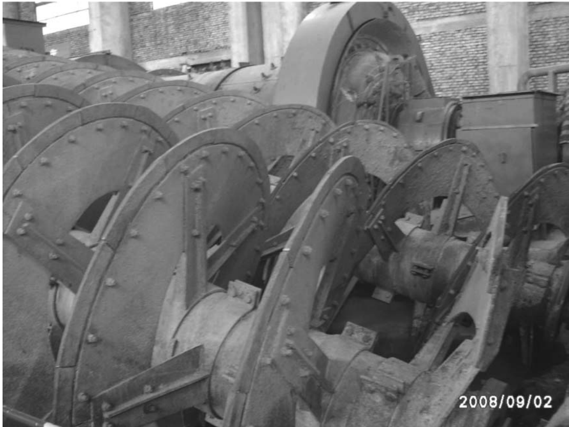
Figure 2.10: Wangji — Phosphate MQG Ball Mill with Obsolete Inclined Spiral Classifiers in the Foreground
